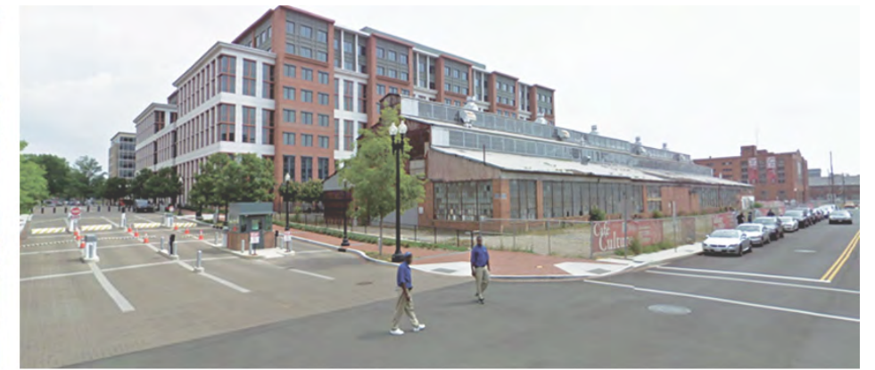
C. ON TINGEY STREET SE LOOKING AT THE BOILERMAKER BUILDING
